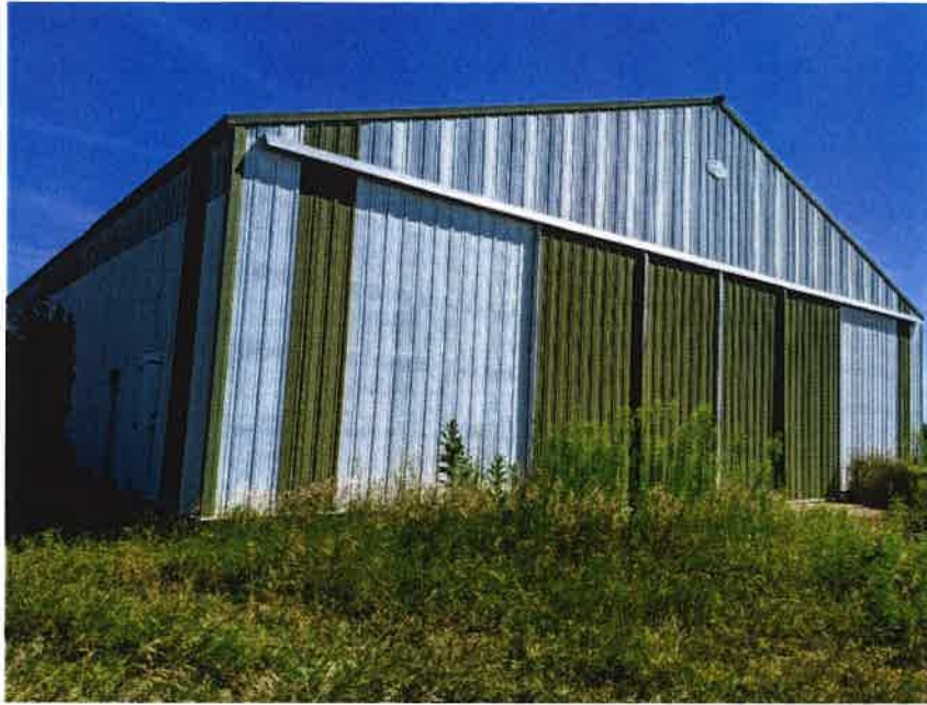
View of the Machine Shed from the SW
