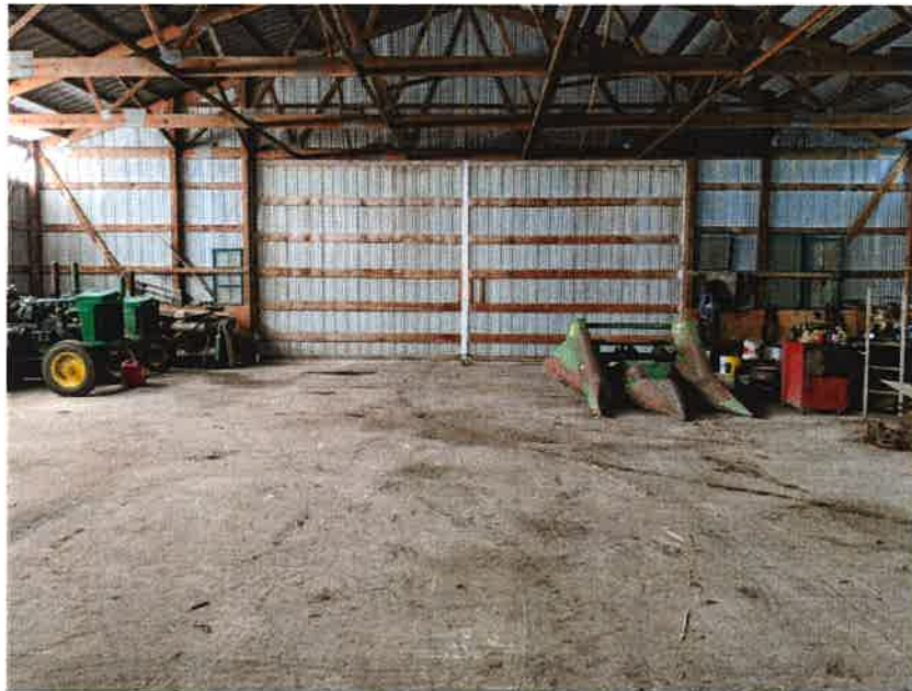
Interior view of the Machine Shed Note the flat grain storage kit
