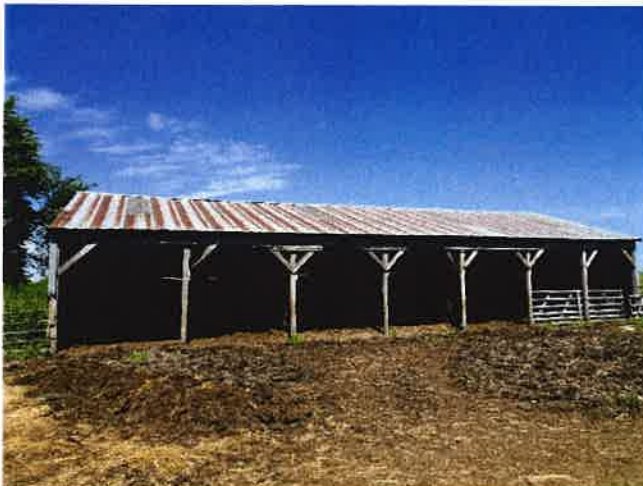
Open-front Cattle Shed
